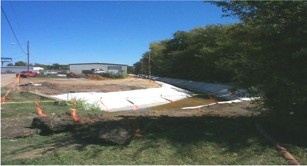
A grout blanket was installed in a stormwater ditch to enhance the drainage along the existing drainage channel.
