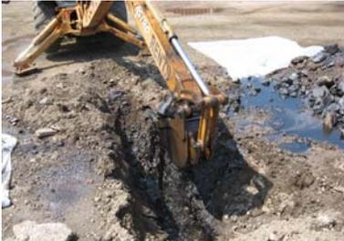
*Geosyntec conducted treatability and pilot tests of the STAR technology to remediate a site impacted by coal tar.*
